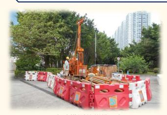
土地勘測的鑚機及相關裝置 ▲ Setting up of drilling rig for ground investigation
