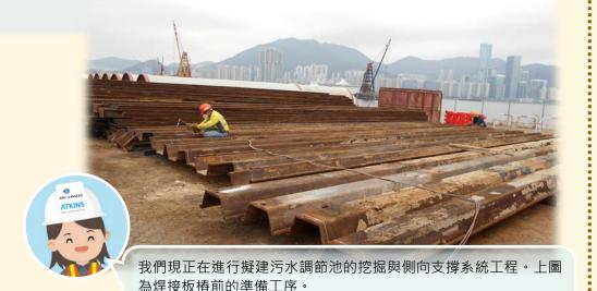
The construction of the lateral support system for balancing tank are in progress. The photo above shows the preparation works for the welding of sheet piles.
