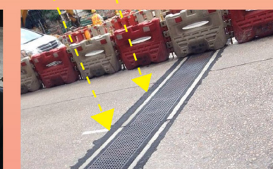
新建路面集水渠 Provision of cut-off drains
