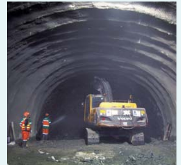
Western Portal – Excavation works for launching tunnel
