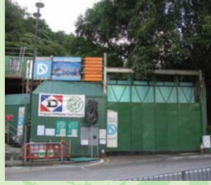
Eastern Portal (Tai Hang Road) – Hoarding has been erected
