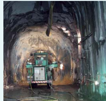
Eastern Portal – Blasting works for launching tunnel
