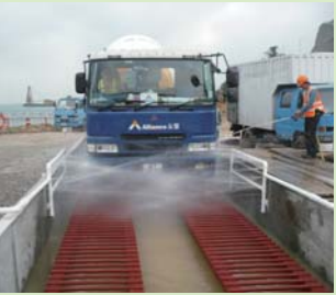
Western Portal (near Cyberport) – Wheel washing facilities
