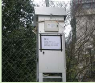
Eastern Portal (Tai Hang Road) – Regular air monitoring
