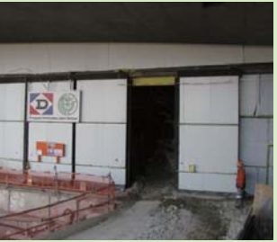
Western Portal (near Cyberport) – Noise enclosure for launching tunnel
