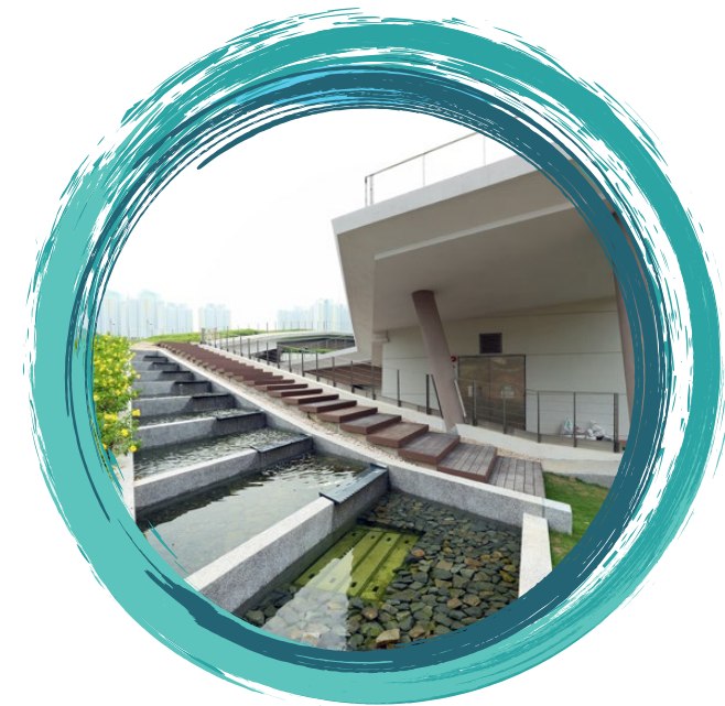
九龍城一號污水泵房 Kowloon City No.1 Sewage Pumping Station
