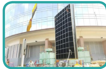
安裝中的一號主泵房新水閘 New penstock inside the Main Pumping Station No. 1 being installed
