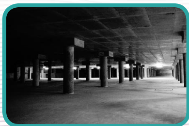
跑馬地地下蓄洪池 Happy Valley Underground Stormwater Storage Tank
