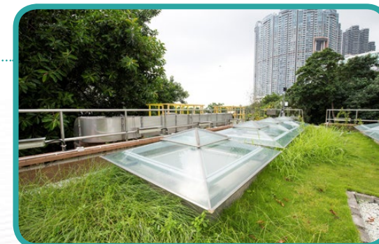
華富基本污水處理廠綠化天台 Roof greening at Wah Fu Preliminary Treatment Works
