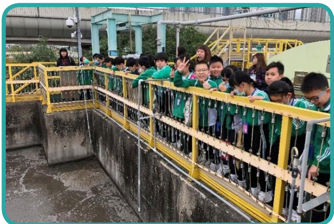
小學生參觀沙田污水處理廠 Primary school students visited Sha Tin Sewage Treatment Works
