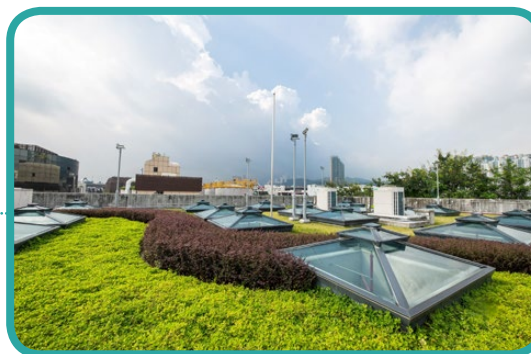
昂船洲污水處理廠化學物儲存樓綠化天台 Roof greening at Stonecutters Island Sewage Treatment Works Polymer Storage Building
