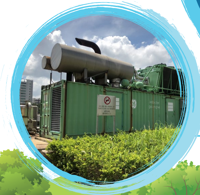
大埔污水處理廠的電熱聯供發電系統 Combined heat and power generating system in Tai Po Sewage Treatment Works
