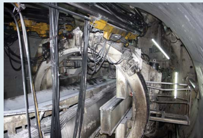
Tunnel boring and mucking out
