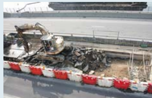
Construction of box culverts underneath Castle Peak Road
