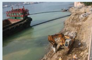
Modification of existing rock armour seawall
