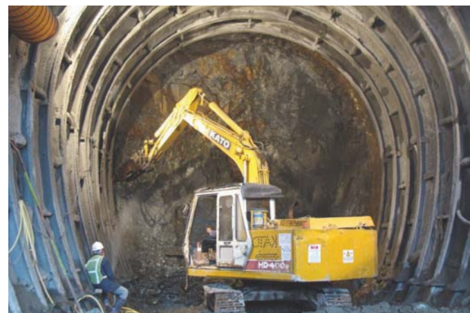
Construction of launching chamber 隧道工程
