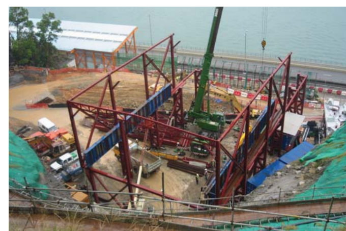
Construction of noise enclosure framework 搭建中的圍封式隔音屏障支架
