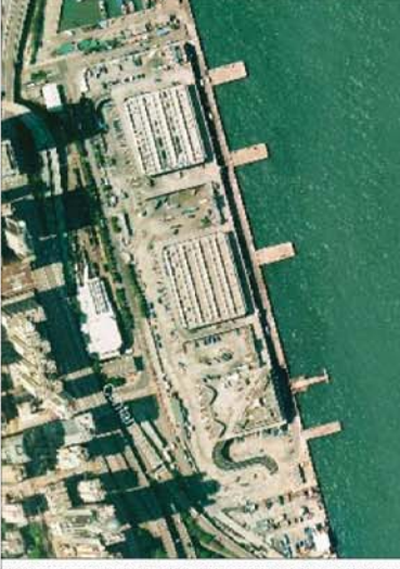
Photo from Baseline Site Visit
