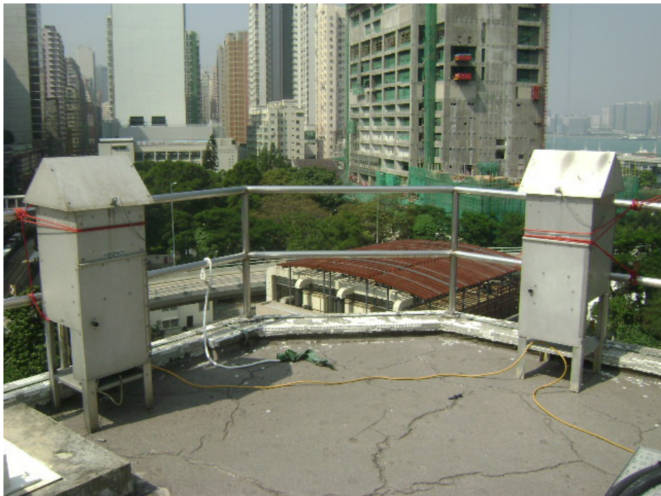
AM2 - Rooftop of Hong Kong & Islands Regional Office, WSD
