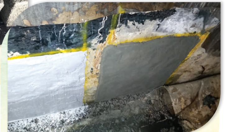
實地試驗中的防腐蝕塗層 Concrete coating in site trial
