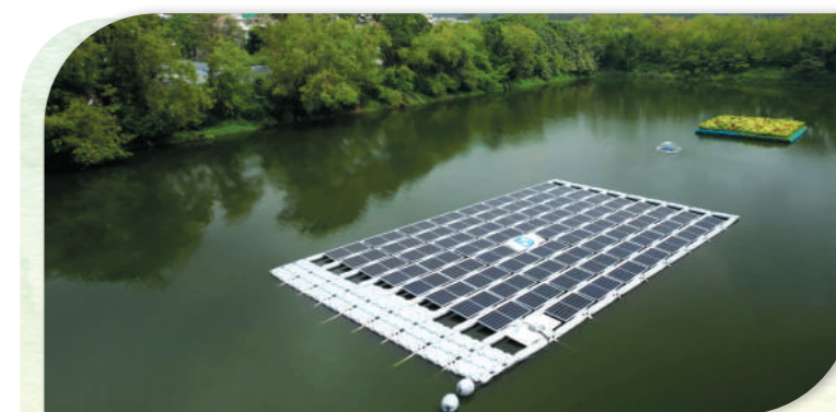
設於新田蓄洪池的浮式太陽能發電系統及生態浮島 Floating Photovoltaic System and Ecological Floating Island at San Tin Polder
