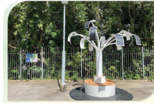
設於新田雨水泵房的太陽能樹 Solar Tree at San Tin Stormwater Pumping Station
