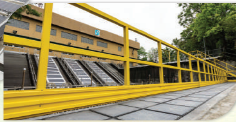
設於新田雨水泵房的可踏式太陽能發電系統 Steppable Photovoltaic System at San Tin Stormwater Pumping Station
