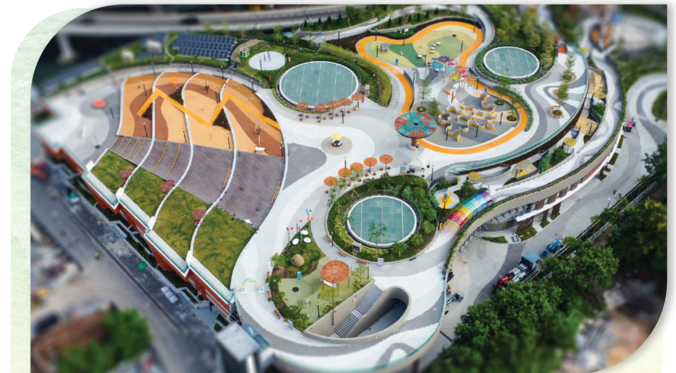
觀塘污水泵房上蓋的園景平台 The landscaped deck built atop the roof of the Kwun Tong Sewage Pumping Station
