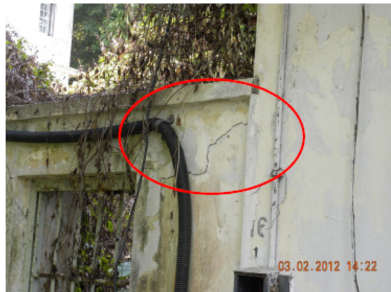
Plate 5 : Condition of an existing crack recorded during the visual inspection survey
