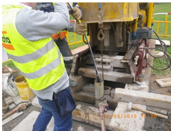
Plate 4 : Installation of Rod Extensometer
