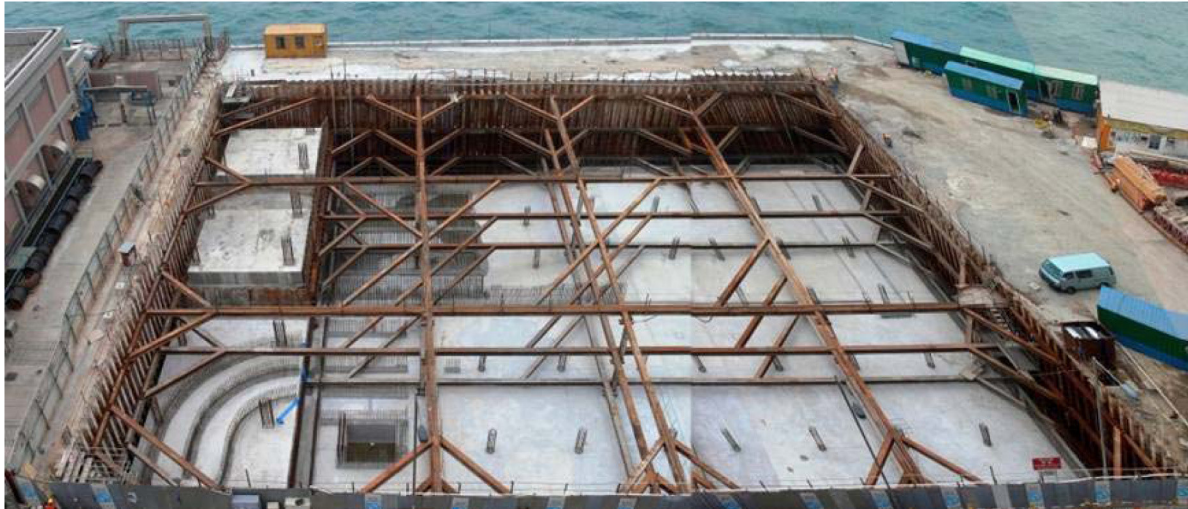
Photo 5: Completed Foundation of Sheung Wan Stormwater Pumping Station
