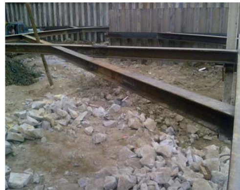
Photo 2: Boulders Exposed in Excavation
