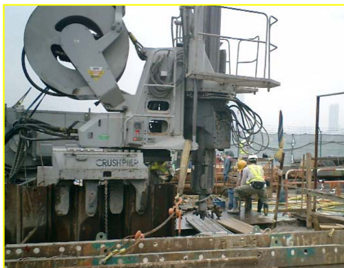
Photo 1: Crush Piler in Operation
