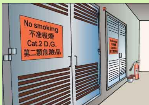
Dangerous Goods Store
