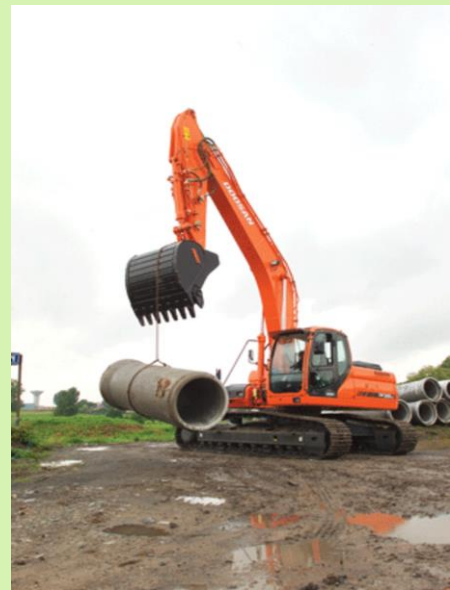
Excavator used for lifting
