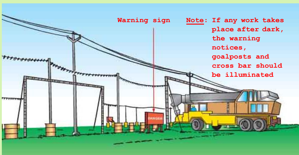
Traffic passing beneath overhead power lines
