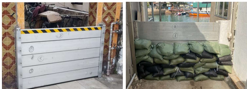
Figure 4 Demountable Flood Barriers in Lei Yue Mun
