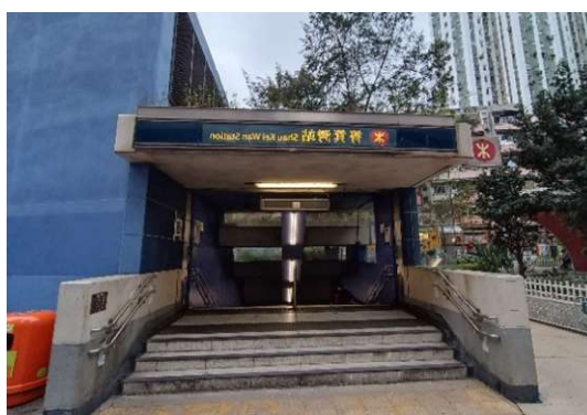
Figure 1 Elevated Entrance for an Underground Facility in Hong Kong
