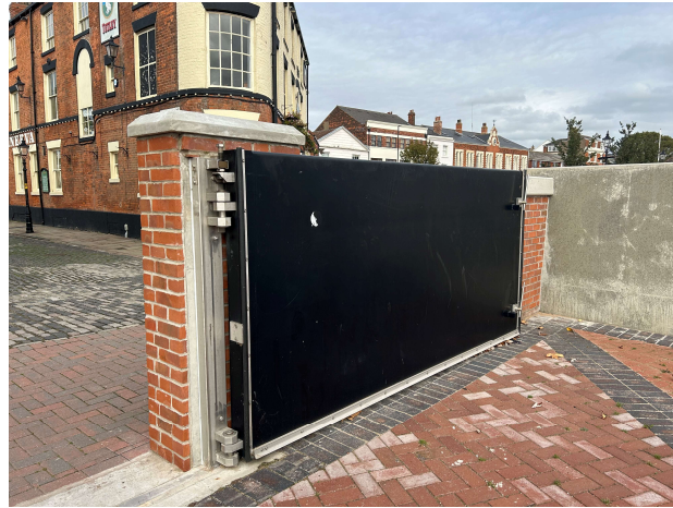
Figure 11 Swing Gate in Hull, United Kingdom
