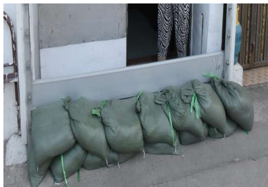
Figure 19 Demountable Flood Barriers with Sandbags
