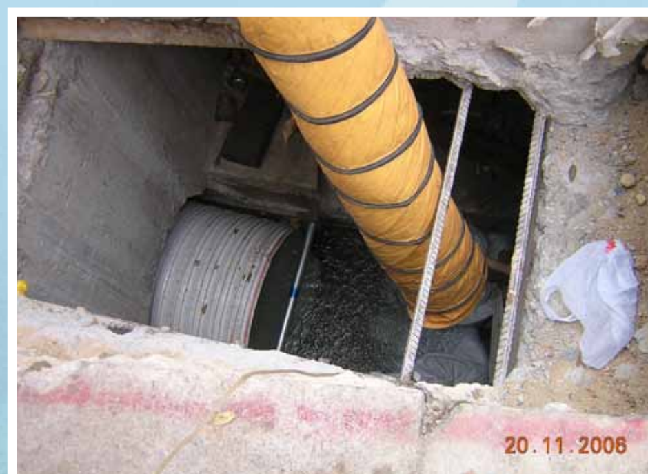
襯管到達下游沙井 Lining formed up to the downstream manhole
