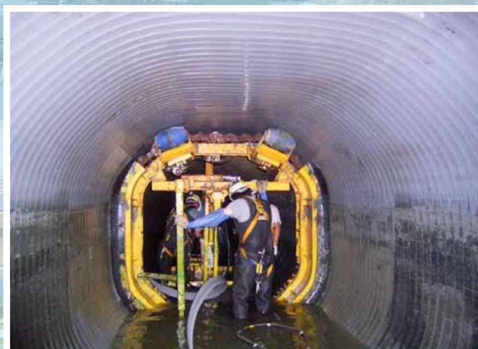
重鋪襯層在大形箱型暗渠內進行中 Lining work in progress inside large-sized box culvert
