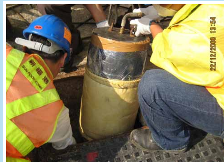
可脹大的卷筒放入沙井內 Inflatable packer being lowered into manhole
