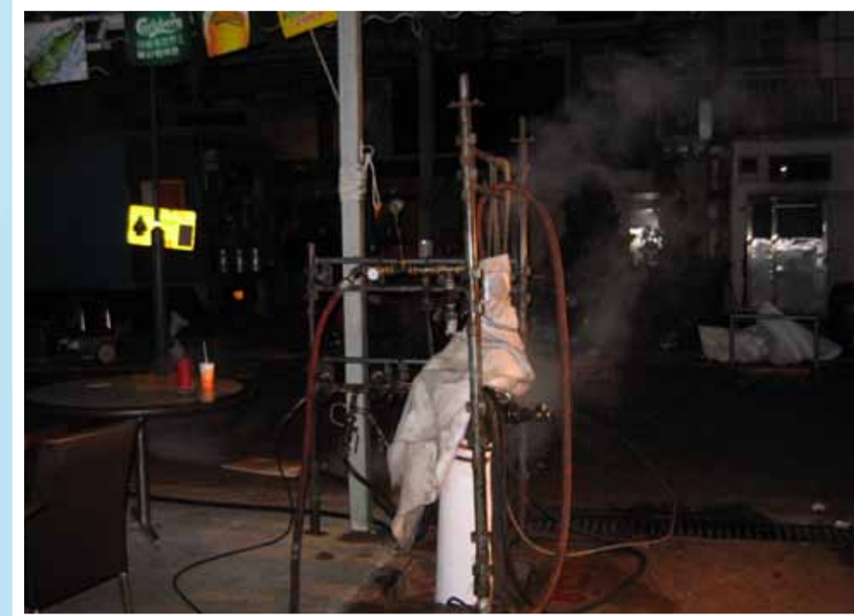
以熱水將套管搪好 Curing of liner by hot water
