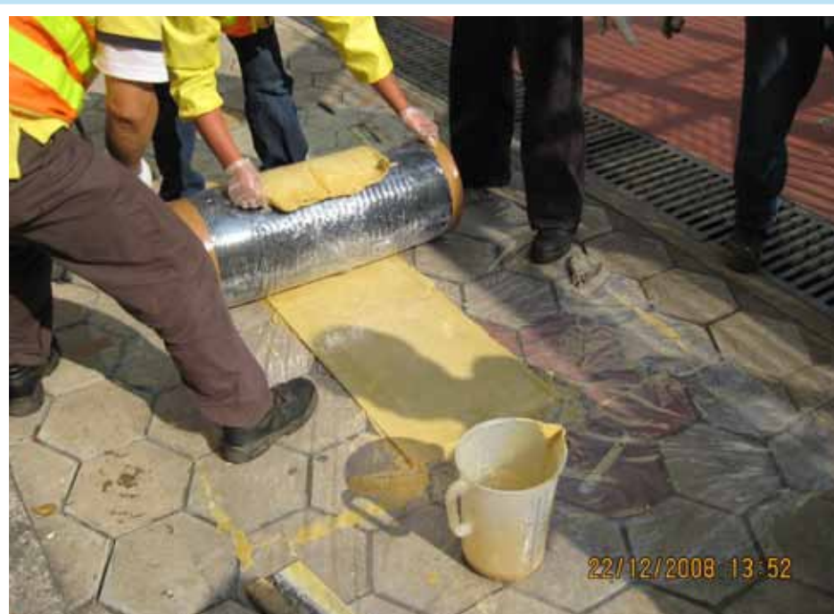
可脹大的卷筒卷上黏附樹脂的襯層 Resin-impregnated part-liner being laid on inflatable packer
