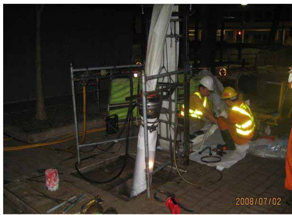
將襯層套管放入渠管 Liner being inserted into pipeline
