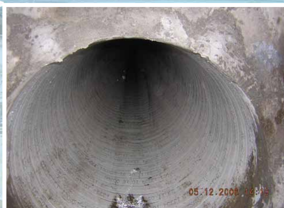
完成的襯管 Completed lining
