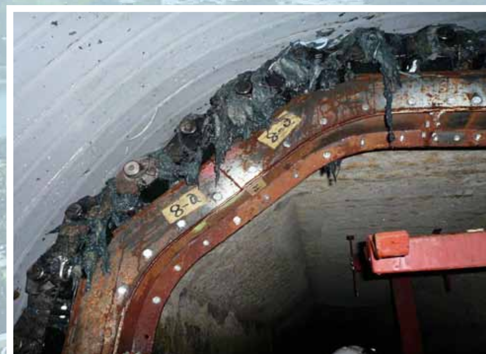
重鋪襯層在大形箱型暗渠內進行中 Lining work in progress inside large-sized box culvert
